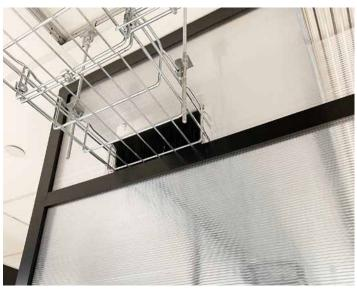
Our proprietary Cool Shield channel is designed to tightly frame the panels for a very effective seal. Panel options (and fire ratings) for our channel include twinwall polycarbonate (E84 Class 1), solid polycarbonate (UL94), CPVC (FM Global) and metal. Most are offered in clear, translucent or opaque.
